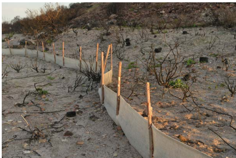
Silt screens help to prevent erosion in an area that is under rehabilitation
