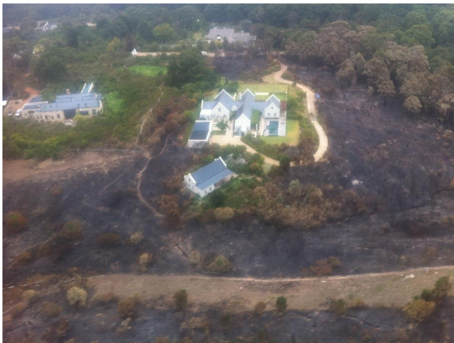
Figure 17: A view of where lawns have provided some defensible space but where woody vegetation has allowed the fire to reach buildings, Muizenberg Wildfire 2015 (Pierre Gallagher, CPFPA)
