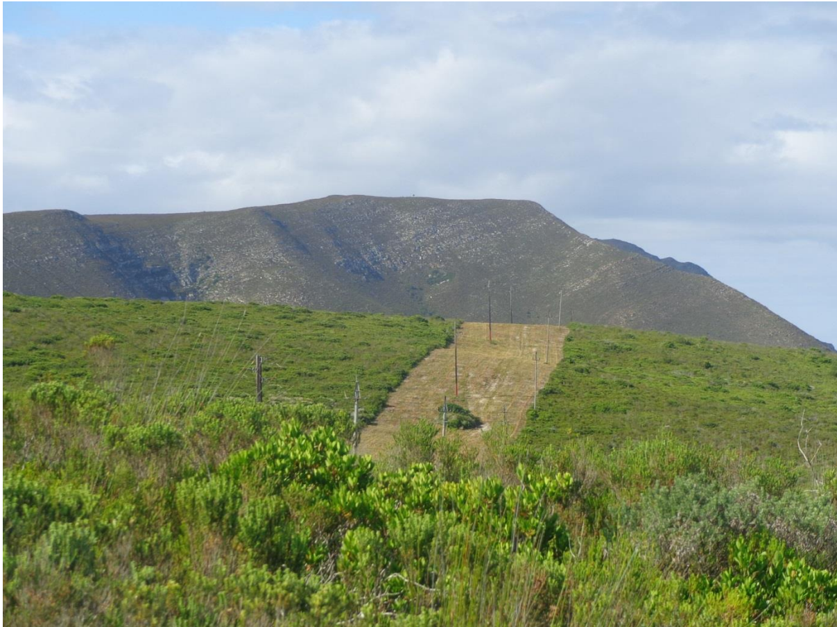
Figure 4: Mowed firebreak running under powerlines in undulating terrain and sandy soils near Gansbaai (Greg Forsyth, CSIR)
